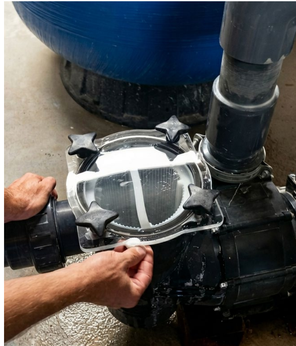
← Repair, Don't Replace When a pool filter lid breaks, a car bracket cracks, or a plumbing component fails — the lab offers an alternative to replacing the whole. A custom acrylic lid, a 3D-printed speaker bracket, a reproduced glove compartment part: small fabrications that solve real problems and extend the life of what already exists. At Fab Lab Armenia, fixing something is as valid a reason to show up as building something new.
